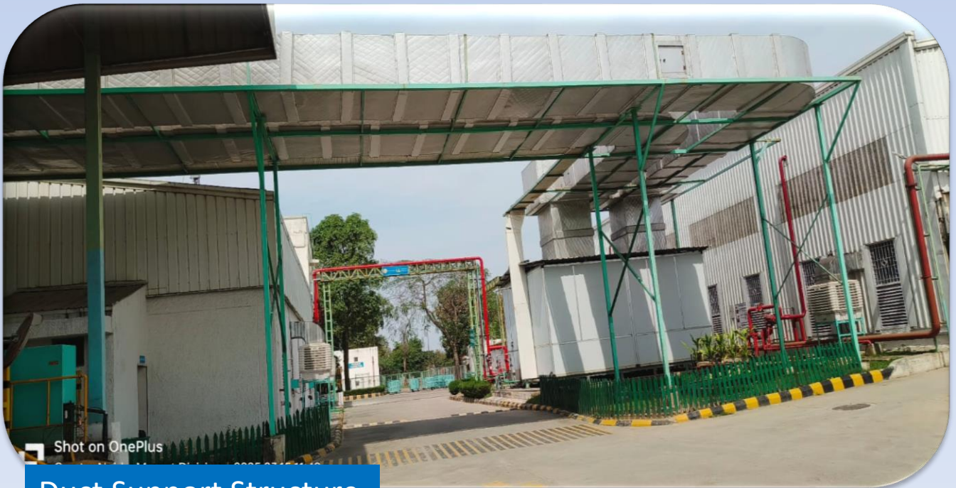
Duct Support Structure
